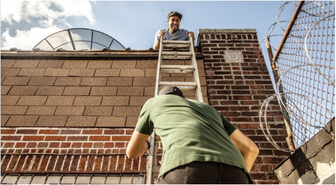
Yamil Lora from The Point CDC in the South Bronx performs site surveys for a new resilient wireless network. Photo: Danny Peralta
